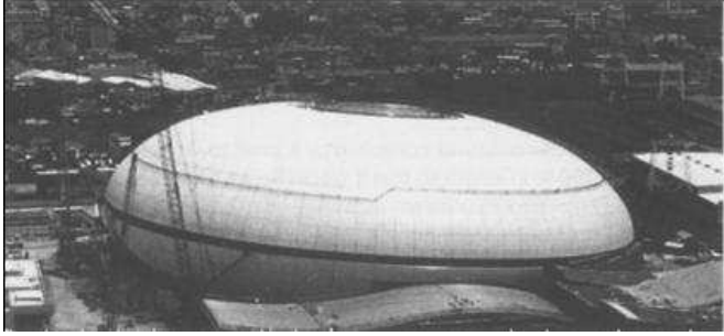
Figure 3: The Namihaya Sports Hall Dome.
