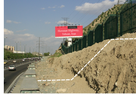
FIGURE 4: Geometry of natural slope behind a retaining wall, Tehran, Iran.
