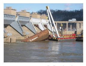
FIGURE 4: Barge impact at Belleville Locks and Dam.
