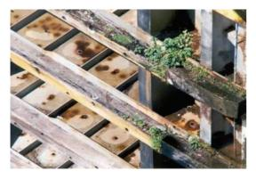
FIGURE 1: Corrosion on a miter gate.
