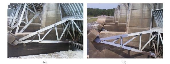
FIGURE 5: Tainter gate with strut arm damage from barge impact before and after repairs.
