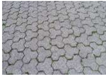
Design of this sidewalk also uses a property that regular hexagons tile a plane
