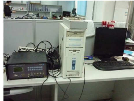
FIGURE 3: Computer of control system.
