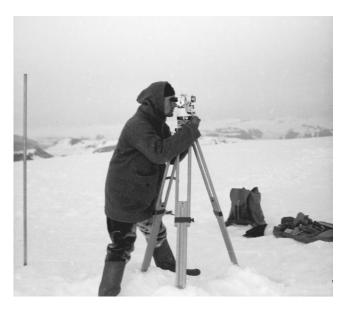
Fig. 4. Making theodolite measurements, Western Greenland 1935.
